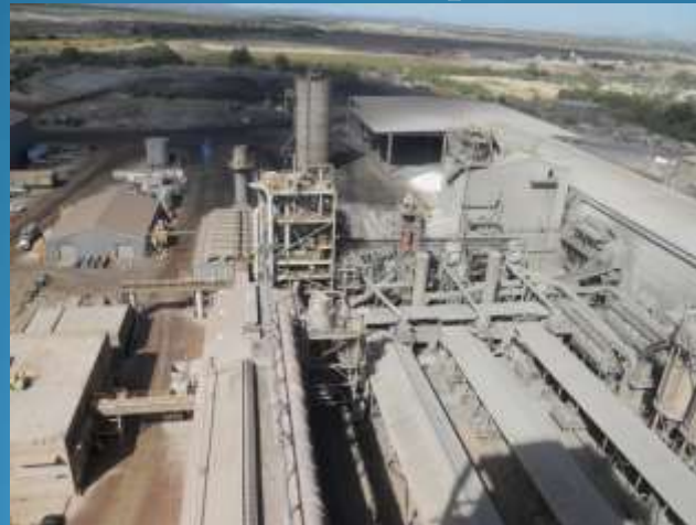
Rillito Cement plant
